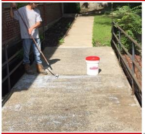
BOND ALL EXTERIOR is an exterior grade, water based, surface bonding agent applied prior to placing new plaster and Portland cement based mixes over masonry, concrete, brick, block, stone, plaster, drywall, wonderboard, precast concrete, wood, tile and EPS board.
