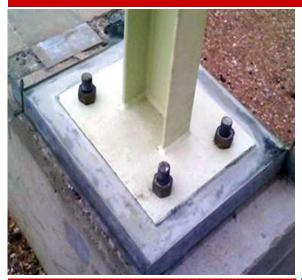
NON-SHRINK GROUT is a non shrink, high strength, non metallic, cementitious grouting compound used for a variety of general construction, grouting and anchoring applications which NON-SHRINK GROUT maintains its strengths at both flowable and trowelable consistencies.
