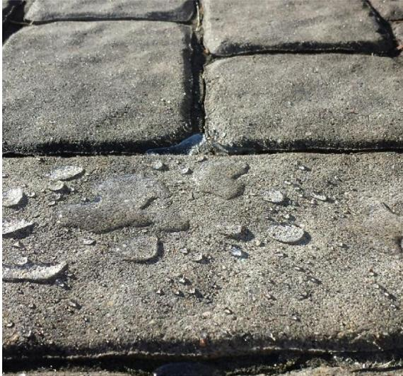
**SILOXANE 12** is an exterior grade, solvent based, clear, deep penetrating water repellent designed to be applied over untreated concrete pavers, brick, block, concrete, stucco, flagstone, granite, natural stone, limestone and bluestone. Breathable, does not form a film or leave a sheen.
