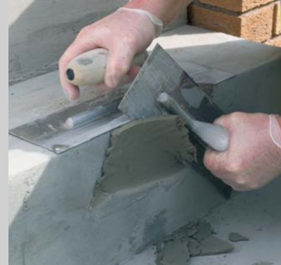
Vertical Patching & Repairs up to 2"
