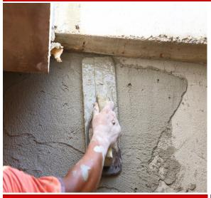
VHO PATCH is a fast-setting, polymer-modified, Portland cement based material specially designed to repair vertical, horizontal and overhead concrete and masonry surfaces.
