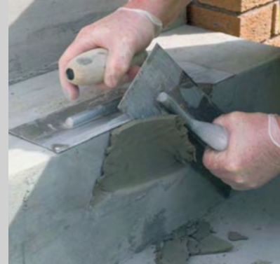
Vertical & Overhead Patching up to 2"
