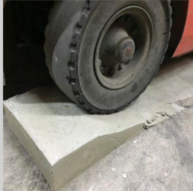
Horizontal Patching & Repairs up to 6"
