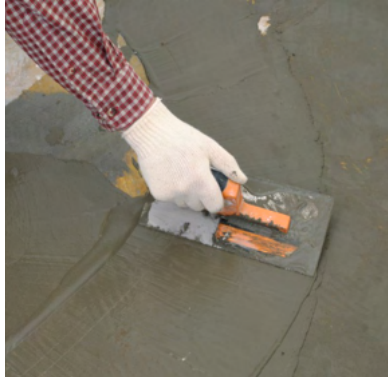
Resurfaces Spalled & Pitted Concrete
